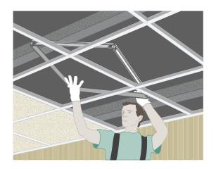
Next, drop the SkyTile into the Elevator.
